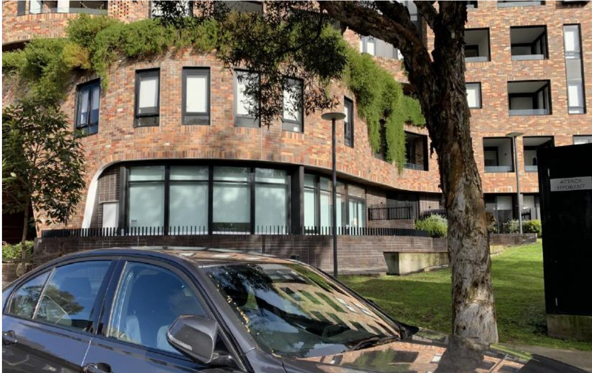
Figure 2: Site viewed from Huntley Street
